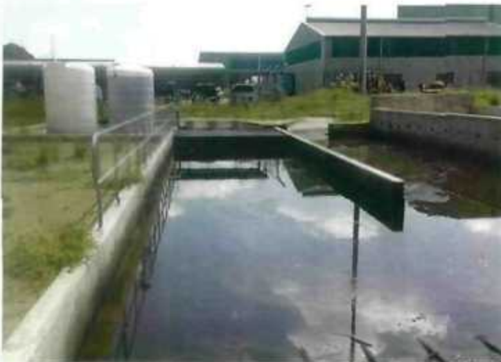
Oily water discharge before the installation of Ultraspin.
