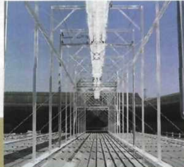
A typical CSP plant based on the Fresnel mirror.
