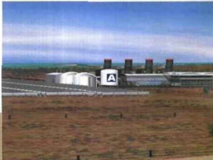
The Elgen plant with a rated capacity of 54 MW. "We are thermal specialists in co-generation projects, one of the few companies that has actually designed and constructed real co-generation plants," claims Matzner.
